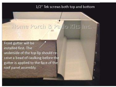
With all your roof panels in place and secured properly, measure the exact length of front gutter assembly you will need. This is the outside edge to outside edge measurement of your panel assembly. If you have more than 24' you will choose a place along the width that will have a butt-splice of the two pieces coming together. This seam will need to be caulked.
